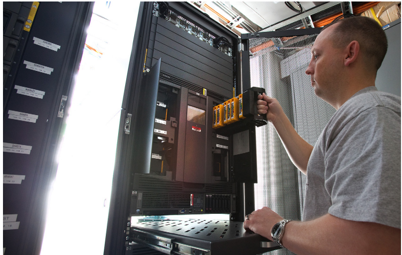
Working in the computer server room.
