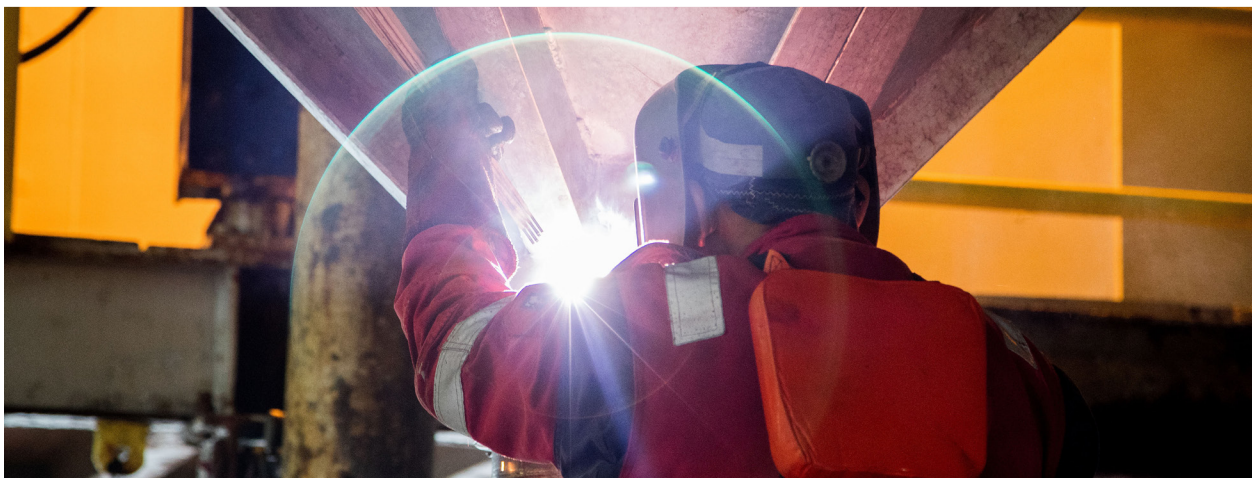
Welding a reentry funnel.
